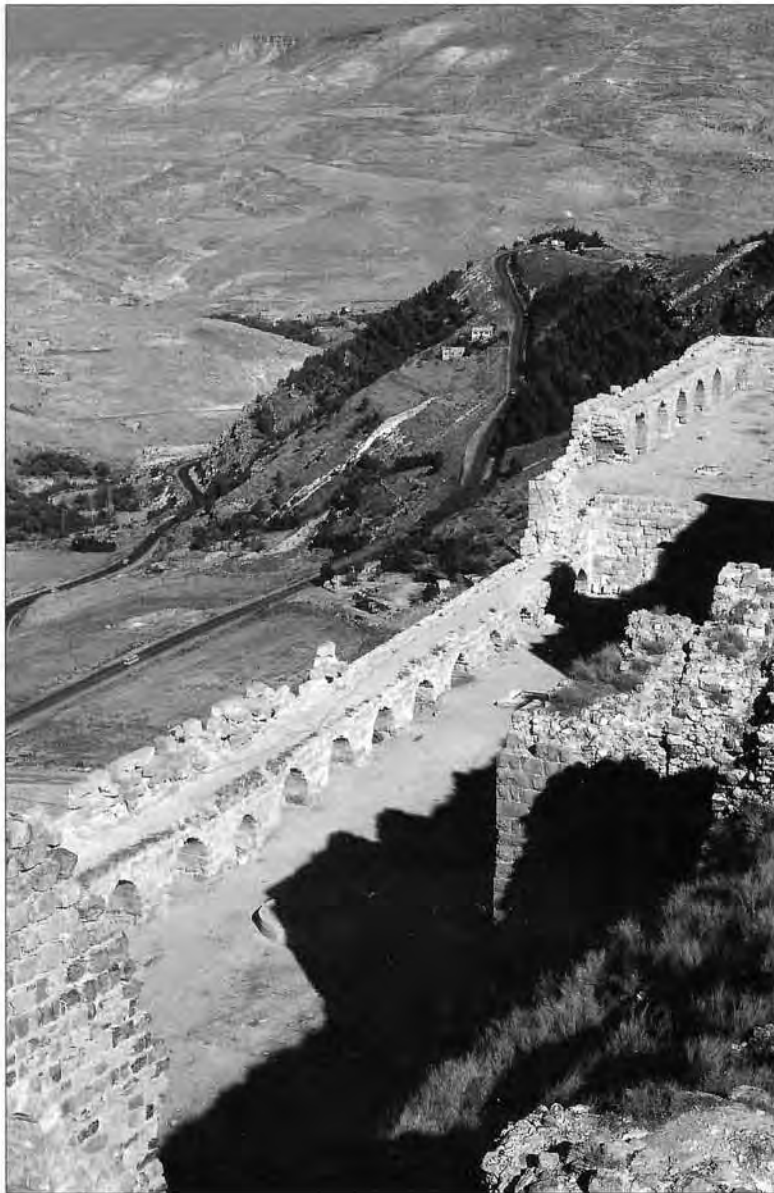
At least two stages in the construction of Karak castle are seen here. In the foreground are the remains of the walls and towers built during the second Crusader phase around 1168. Beyond and below it is a massive barbican dating from the Mamluk era in the late-13th and 14th centuries.
